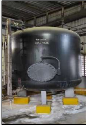
11.1.6 Caustic soda storage tank
